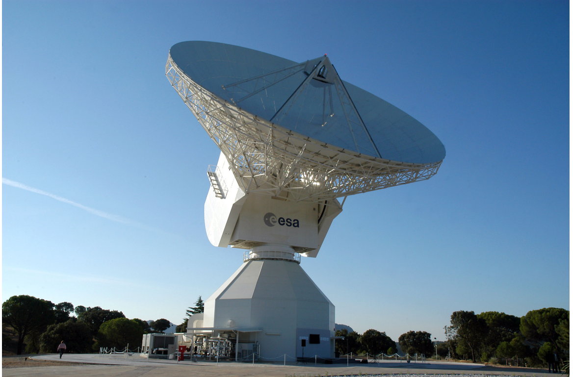
Figure 2.10: ESA’s 35 m-diameter deep-space dish antenna, DSA-2, is located at Cebreros, near Avila, Spain, as part of the ESTRACK network. From [47].
