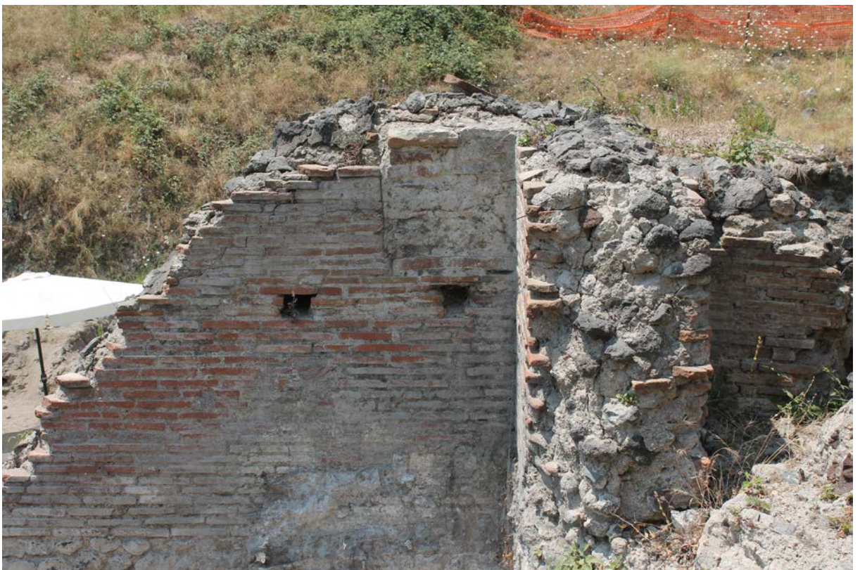
Figure 9 Springing of the probable cross vault in room C.
