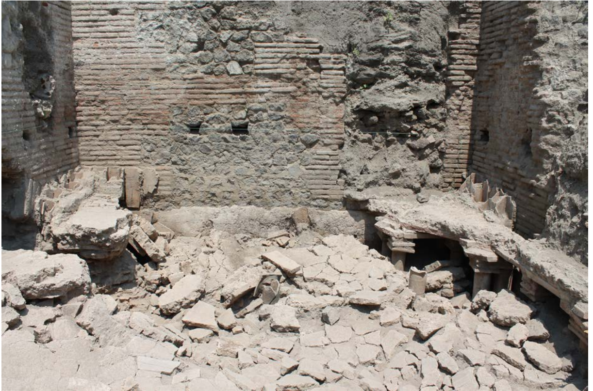
Figure 8 Collapsed floor in room C, showing suspensurae and tubuli.
