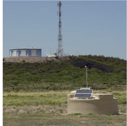
Figure 3.2: A picture of an SD station and FD building. Each station has its own solar panel with battery and communication antenna. There is also the antenna close to the nearby the FD building.
