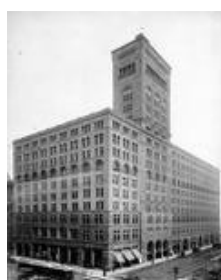
obr. 6 Auditorium Building, Chicago Dankmar Adler, Louis H. Sullivan, (1886 - 1890)
