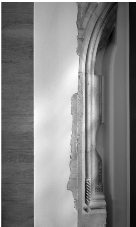
FIG. 7: Prague Castle, the former palace of Archduke Ferdinand by the White Tower. Part of a window (or door) on the eastern end of the palace's northern facade on the first-floor level (© Petr Chotěbor).
