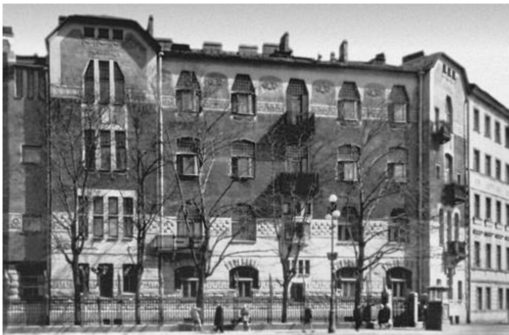
Fig. 4. The house of Fedor Lidval at Kamennoostrovskiy prospect, 1-3, constructed in 1899 – 1904.
