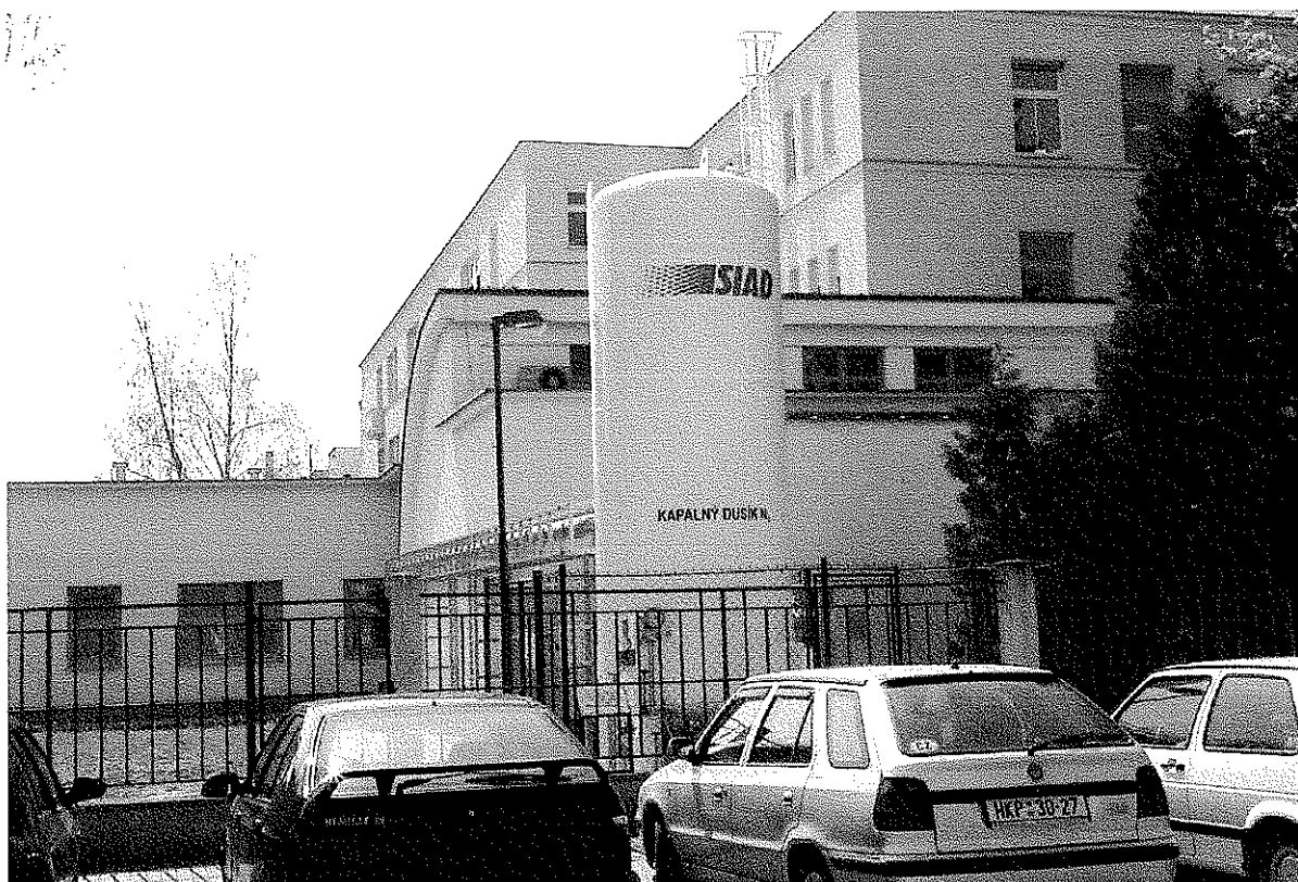
Figure 1: The outer view of the Tissue Bank, University Hospital, Hradec Králové. The outer tank can contain, maximally, 4,000 kg of liquid nitrogen. Critical parameters, i.e. the liquid-nitrogen weight and the pressure inside the container, are continuously monitored and recorded. The container is connected by an insulated tubing to the cryostorage rooms and cryopreservation laboratory (front right). The clean-room facility, with the critical processing-areas, is situated in a building seen at front – left. The high building behind the bank is the Department of Gynaecology and Obstetrics.
