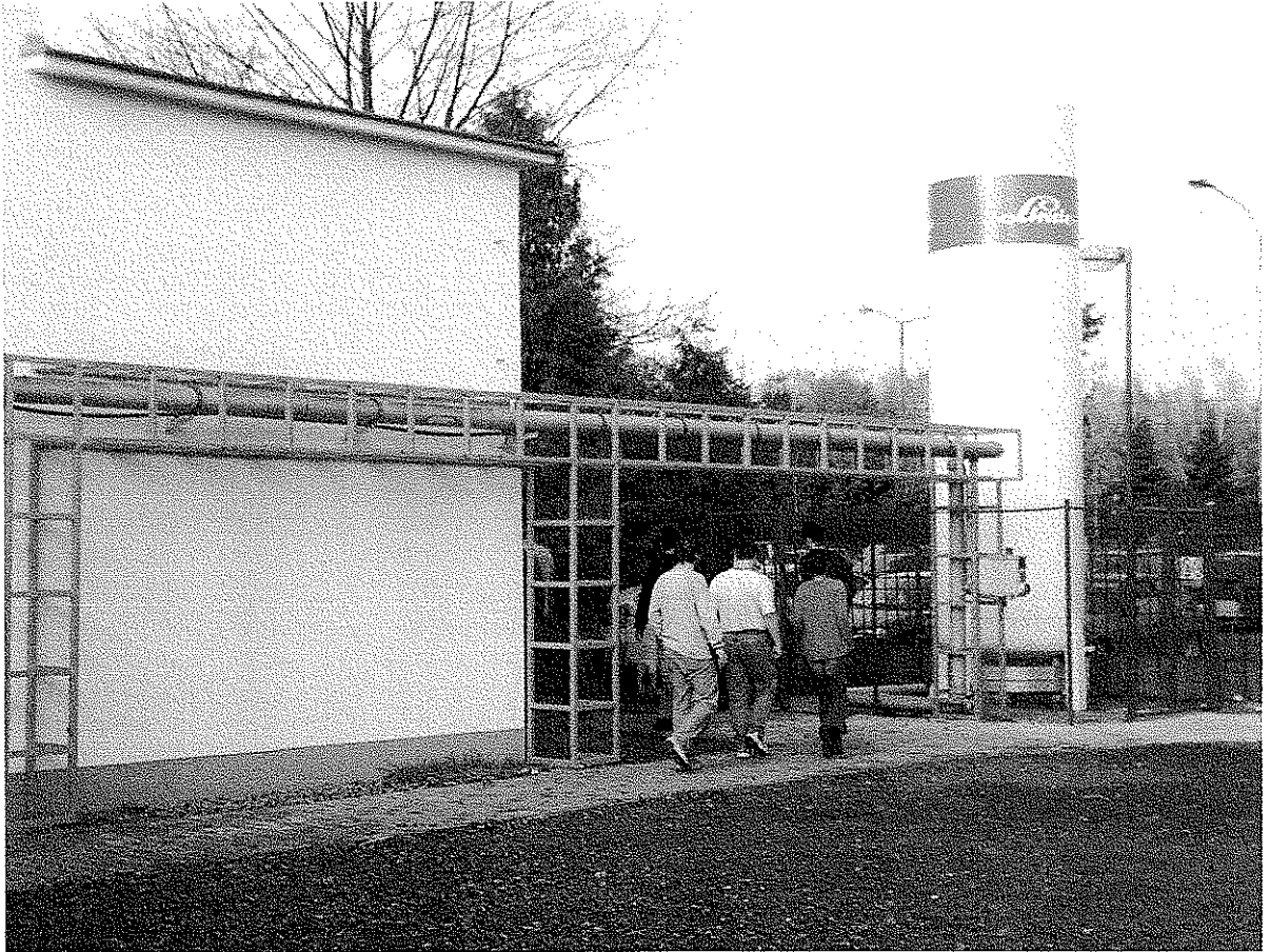
Figure 3: The insulated tubing connects the outer liquid-nitrogen container to the cryobank. The metal construction around the tubing lowers the possibility of mechanical damage.
