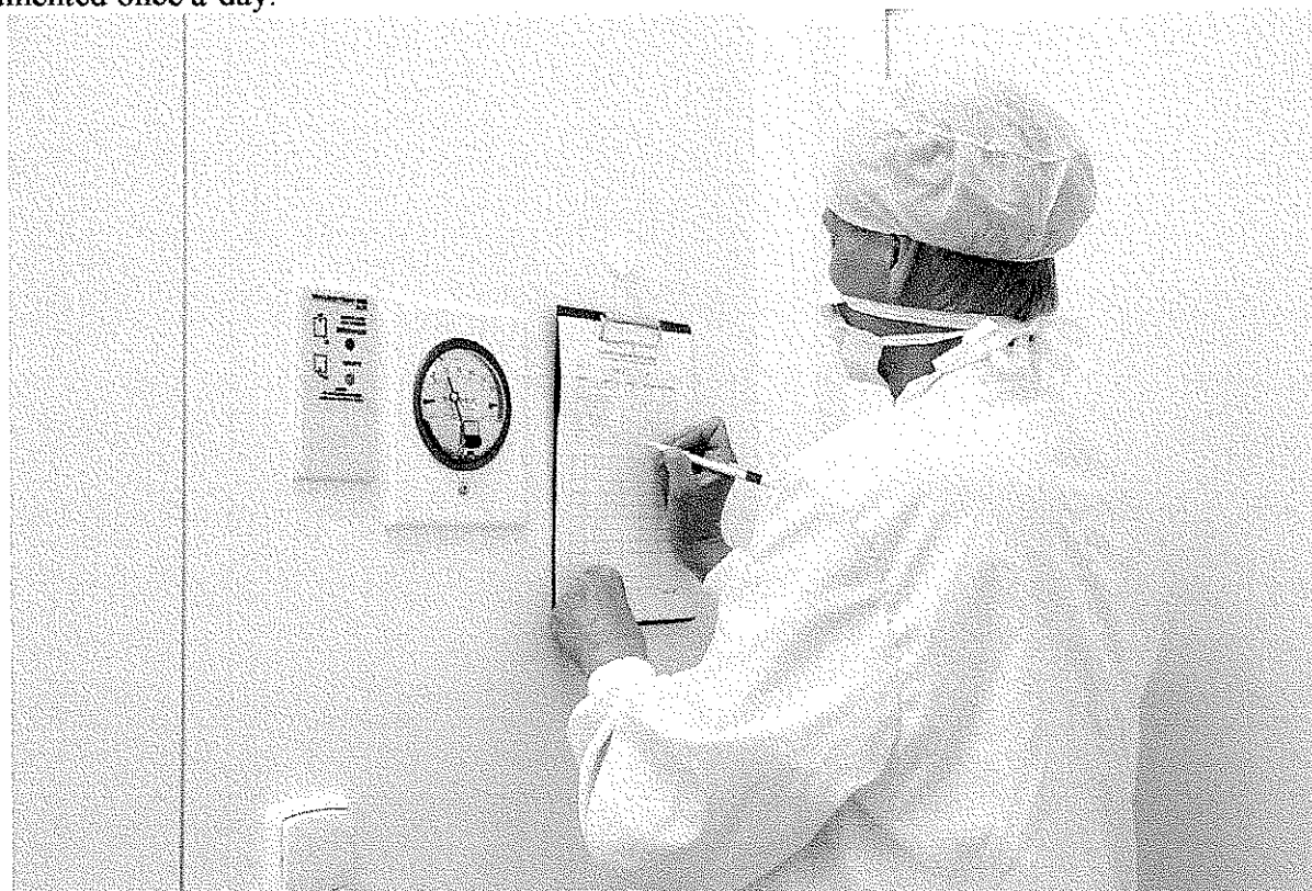
Figure 11: Differential-pressure manometers are placed at entrances to personal corridors. Here, a clean-room operator, wearing a suit used for Grade C areas, enters the corridor into a Grade B area. Each entry is registered.
