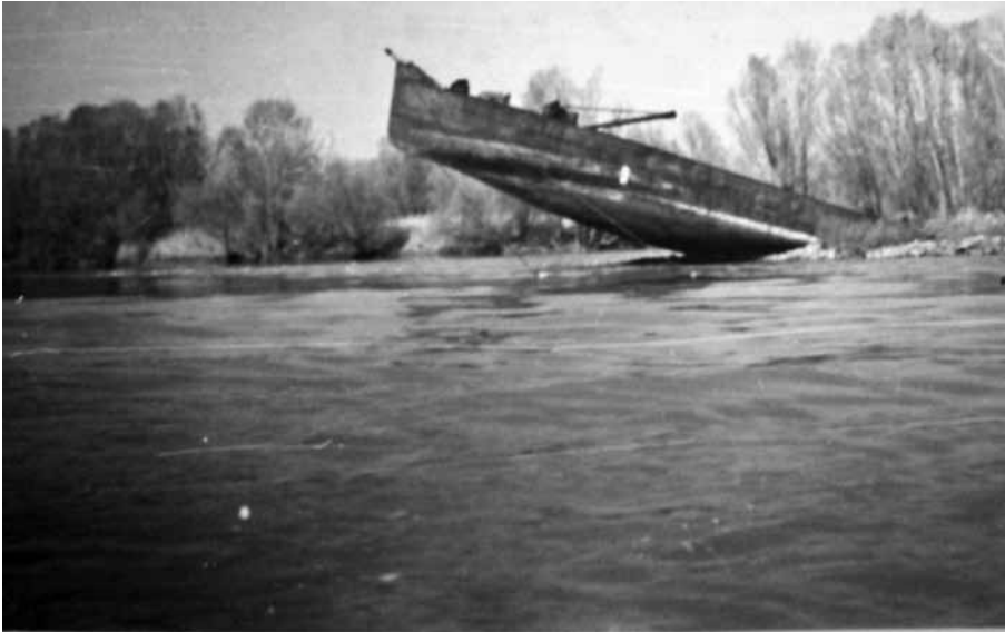
Figure 4.1 – The war negatively affected the state of waterways in Europe. Necessary repairs required enormous efforts, but simultaneously opened the door to bold reconstruction schemes. The picture shows a ship-wreck on the Danube, which remained in this position long after the war ended, well into 1946. Source: NAČR, CPU, b. 96.
