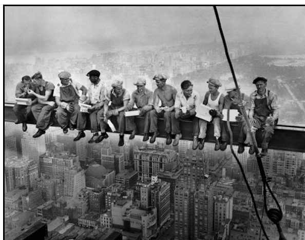
Obr. 13 - Construction Workers Lunching on a Crossbeam 17
