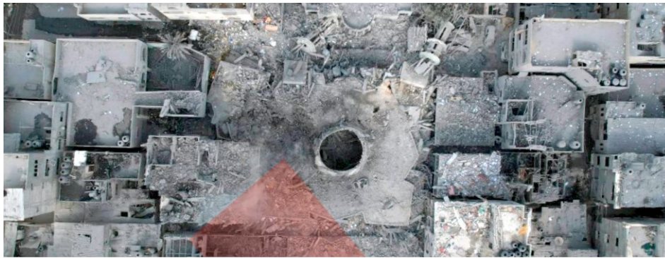
Figure 13: Georeferenced drone footage of Ahmed Yassin mosque post-airstrike (October 9) with 20-meter cluster-based change mask overlay
