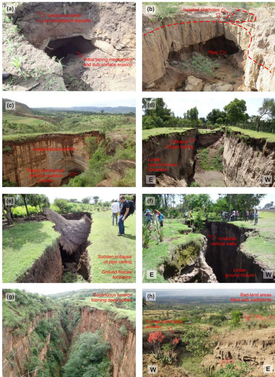
FIGURE 7 Field photographs of successive stages of ground fissure formation: (a) isolated sinkhole in unconsolidated deposits and initial piping mechanism associated with sub-surface erosion (location); (b) isolated sinkholes interconnected by a pipe (Leku); (c) large-scale sinkhole and pipe in lower part (Boditi); (d) linear north–south (N–S) trending ground fissure formation associated with ceiling collapse (southwest of the town Awassa); (e) destruction of farmers facilities due to sudden collapse of pipe ceiling and ground fissure formation; (f) linear N–S trending ground fissure with unstable steep walls (Leku); (g) continuous erosion around the ground fissure forming deep gullies (Boditi); (h) later fluvial-dominated erosion and ‘bad-land’ formation (southwest of Awassa town) [Color figure can be viewed at wileyonlinelibrary.com ]
