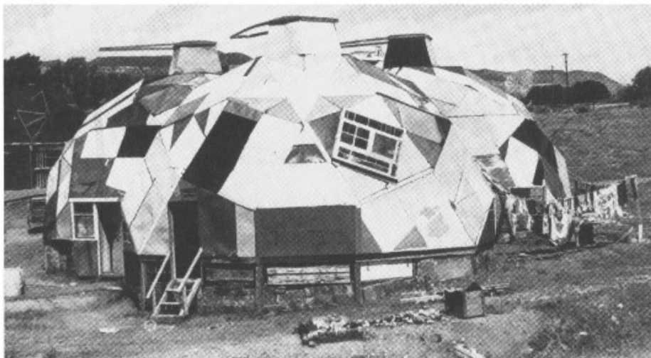
Drop City – geodesic dome from scrap metal, after 1966. In: Miller 1992.
