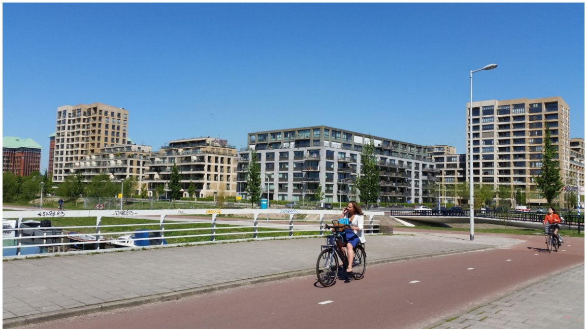
Fig. 19: Andreas Ensemble in Amsterdam Nieuw-West
