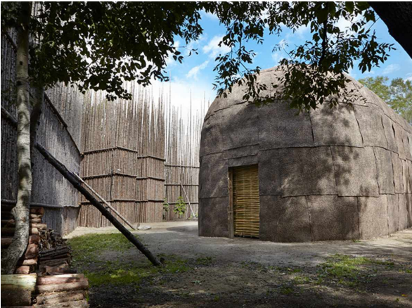
Figure 7: Replica of an Iroquois longhouse. Long and narrow, this bark-covered single-room structure used to host several families. The longhouse of the museum is smaller than the actual traditional buildings, but the structure includes storage spaces and fire pits. © Québec Original
