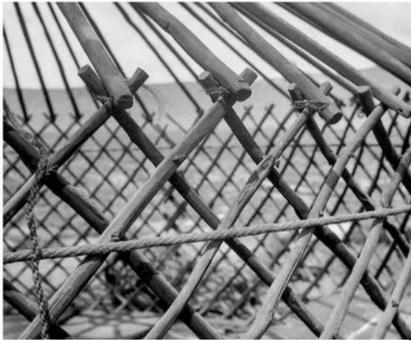
Fig. 21. The roof poles rest on the ‘saddles’ at the top of the trellis wall. (Braae 2017, 215.)
