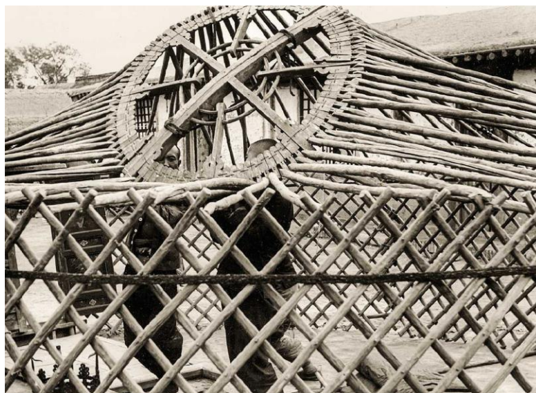
Fig. 48. Roof wheel of the sarchinag type, 1938. National Museum of Denmark Digital Collections. (Photo: Kaare Grønbech.) Courtesy of the National Museum of Denmark. https://samlinger.natmus.dk/ES/asset/354465
