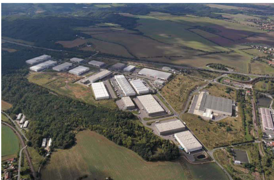
Fig. 3 – As Rudná is located very close to Prague, many new warehouses and service centres were established here. There has been a lot of development in the whole territory since 2000. Photo by J. Pištěk.
