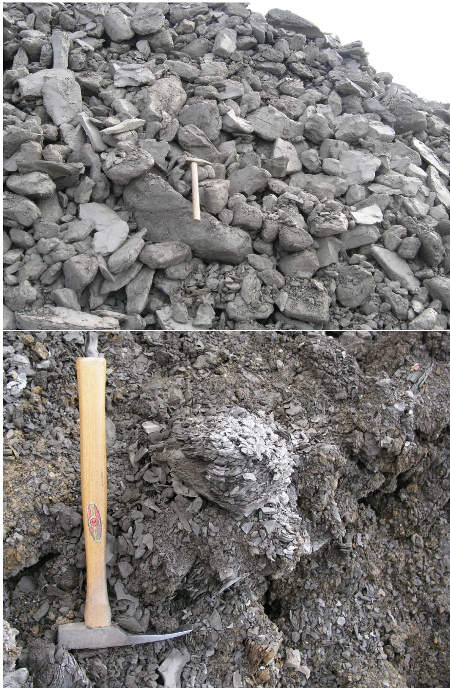
Figure 5.7: Clay fill just after filling (top); Surface of the clay fill exposed about 6 months (bottom), both from Břlina mine.
