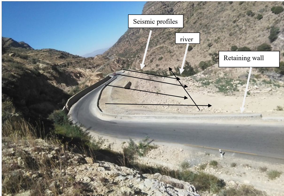
Fig.5. Seismic profiles in Adi Mesnu Landslides
